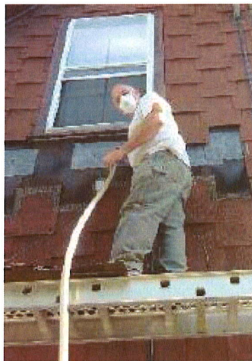
Bill Newell preparing to dense-pack walls with blown-in insulation.
